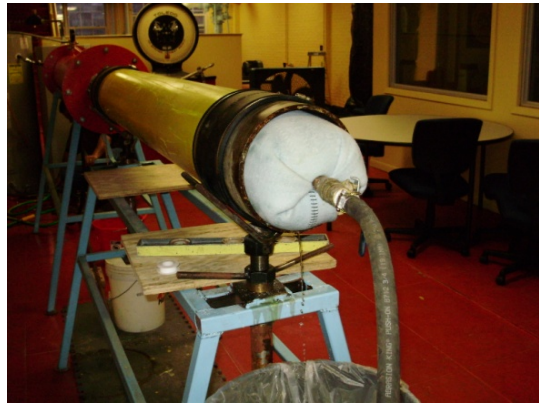
Liner cure under pressure
