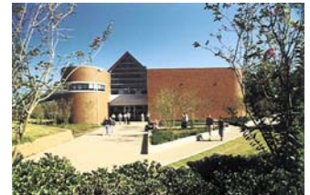
Institute for Micromanufacturing Louisiana Tech University Ruston, LA
