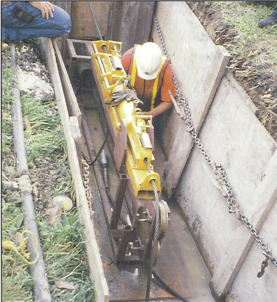
The PIM Corp. performed a pipe bursting demonstration in Houston.
