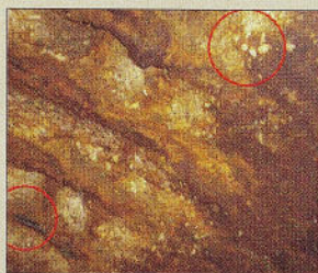
Above: 900-mm concrete sewer pipes that experienced severe MIC;
