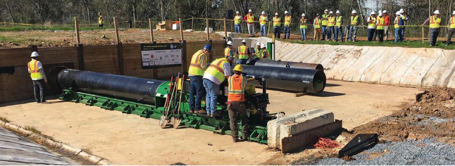
Above: At the auger boring field facility, students were first instructed individually to get better understanding of the equipment. Any student could operate the machine and experience boring, but first had to go through a short orientation and hook up to the shutdown tether. The instruction later continued still in small groups for better hands-on experience. Left: Fluids lab led by Frank Cannon and Ed Anderson of Baroid Drilling Fluids was educational – and fun. Here, Cannon was playfully but effectively illustrating the power of lubricants. Below: Brian Dorwart instructing one of the classes in the contractors' track.
