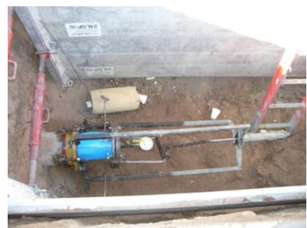
Liner Tensioning Device
