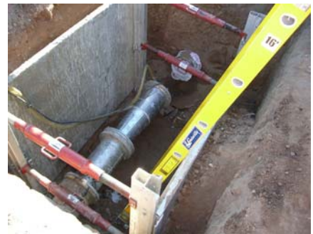
Swab Insertion Chamber
