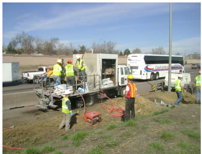
MainSaver Installation under I-25 in the City of Thornton
