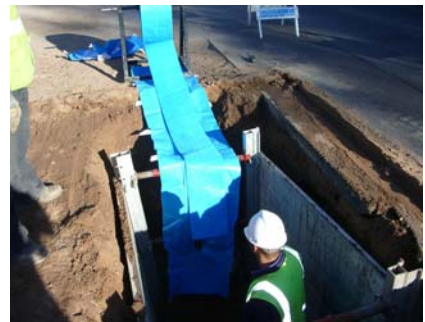
Inserting tube into host pipe
