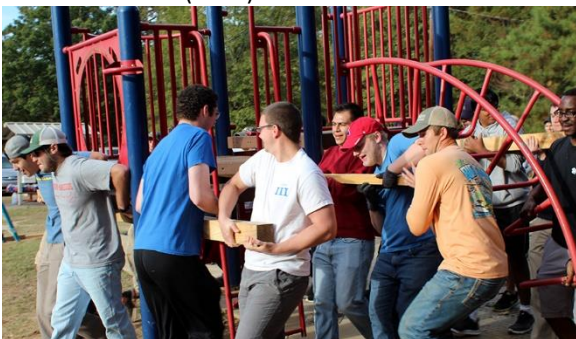
Moved a Play System across the Road at Mayfield Park with Construction Engineering Technology Students and Bulldogs Without Borders (2016)
